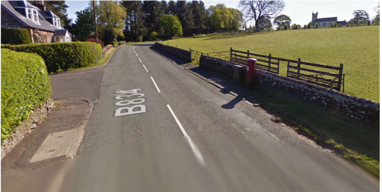
Figure 2.1: Intermittent Footways Both Sides of Station Road
